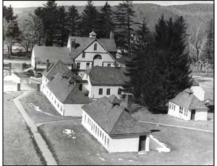
The Craft Shop is left foreground, the Print Shop right. The Coop is the L-Shape building beyond the Craft Shop.
