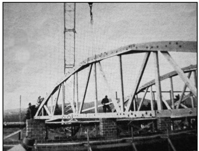
Giant 'cherry-picker' swings Gym roof trusses. (1949)
